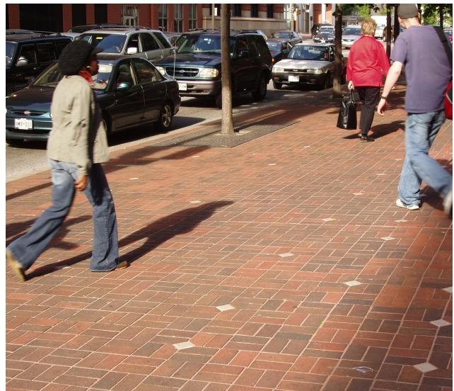
Photo 4 Clay Paver Sidewalk in Basket Weave Pattern
