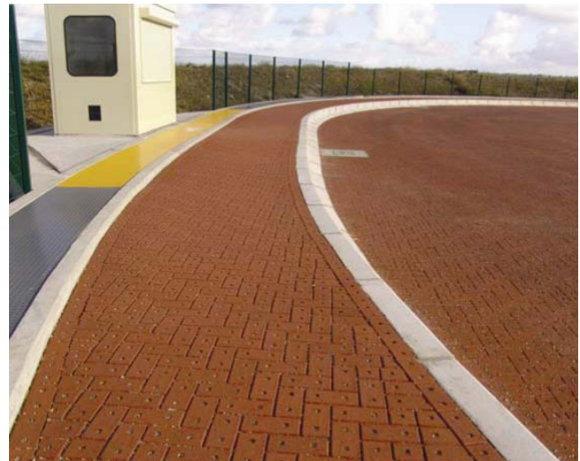
Photo 6 Permeable Clay Pavement
