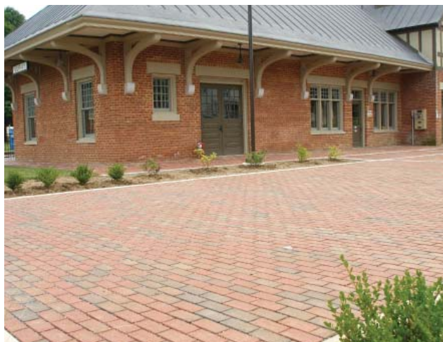
Photo courtesy Pine Hall Brick Company, Inc.
