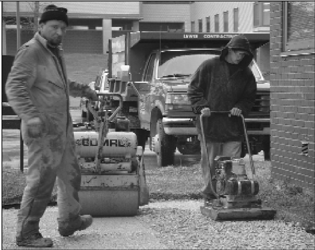
Figure 12: Compacting Near Edge
