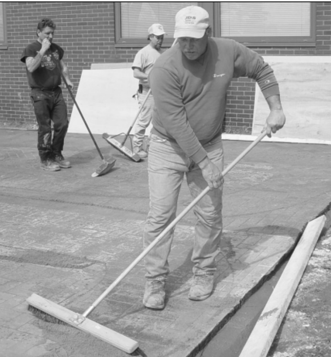
Figure 16: Sweeping Joint Sand
