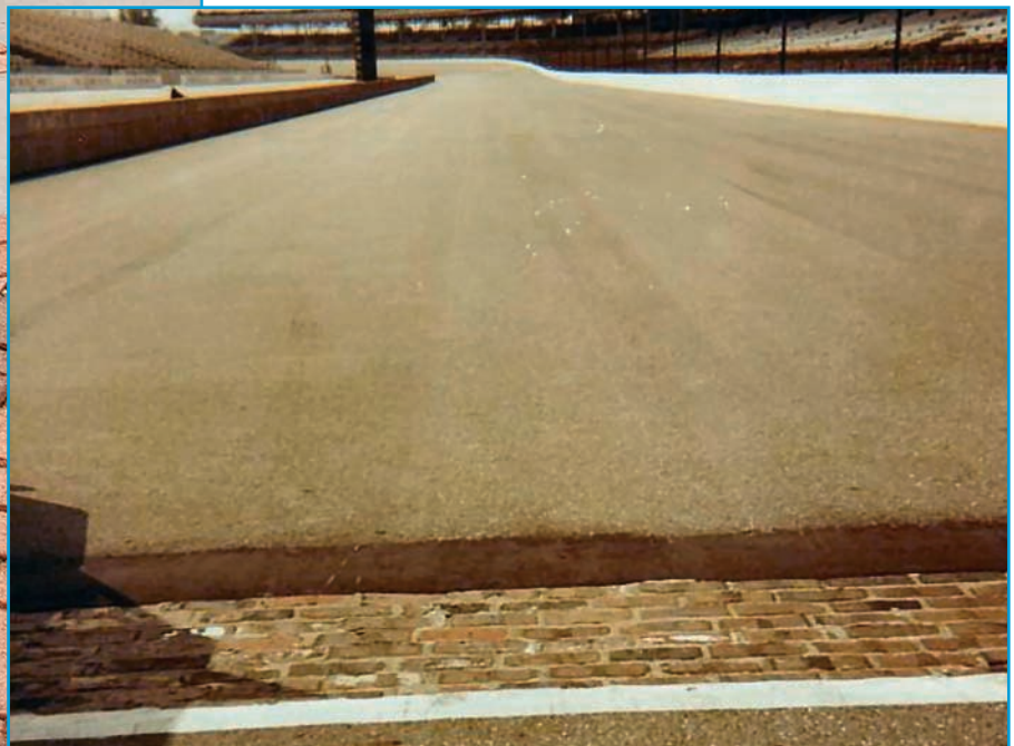
It is interesting to note that the Indianapolis Motor Speedway was surfaced with more than 3 million clay pavers before it was covered with asphalt. The original pavers still stand at the start/finish line of the track as shown.
